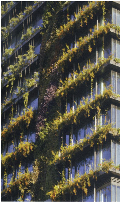
Figure 3. The vertical gardens maintained by the hydroponic system.
