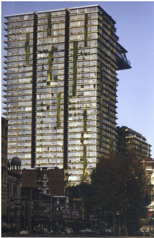
Figure 11. Deep vertical slots carved into the building to allow light and air.
